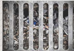
SEWER PLUMBING SERVICES
